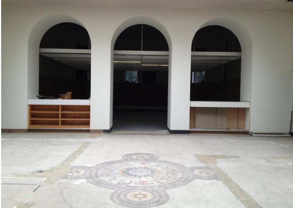
Figure 4. Carnegie Library Interior as Found by Koning Eizenberg
