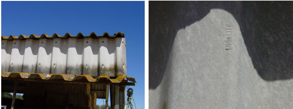
Figure 4. Roof of an agricultural building and detail of the fibre cement sheet with the “Lusalite” logo
