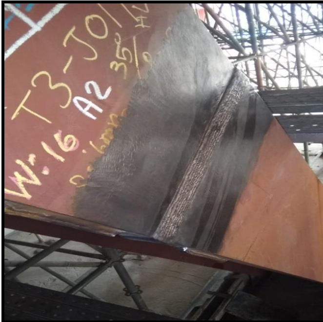
Figure 6. Welding 3G Position for Heavy Thick Plates
