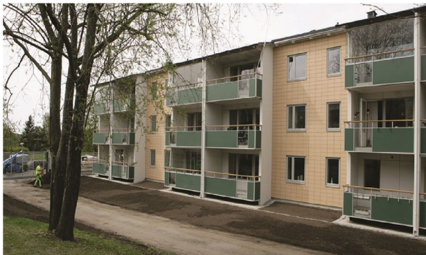
Figure 4. Brogården Project, Sweden
