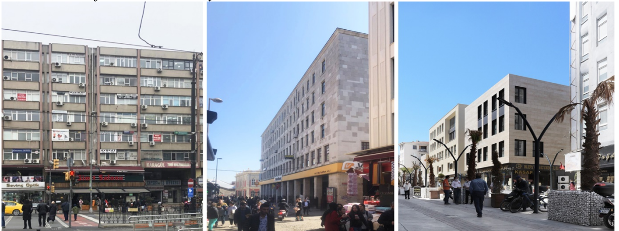
Figure 5. Bureaus on the Upper Floors: Karagul Is Hani, Istanbul; Vakif Is Hani, Istanbul, Merzifon Is Hani, Amasya
