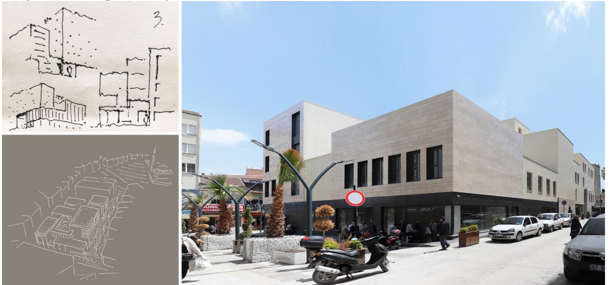
Figure 14. The Sketch for Minimization of Stone on the Façades and the Fragmental Composition of Stone and Stucco
