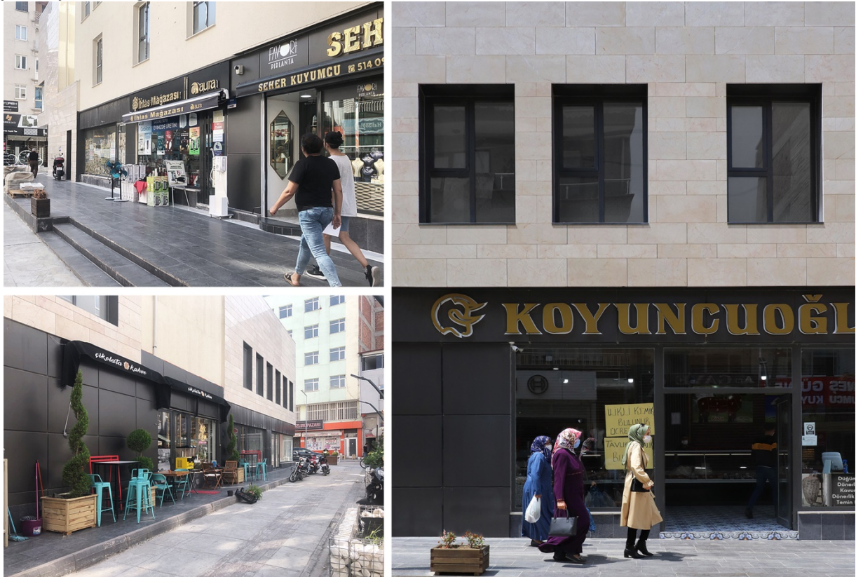
Figure 15. Various Types of Shops and Active Shopfront Interface on the Ground-floor of Building
