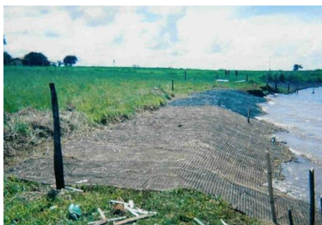
Figure 3a. Implementation of Gabion Mattress in 2002
