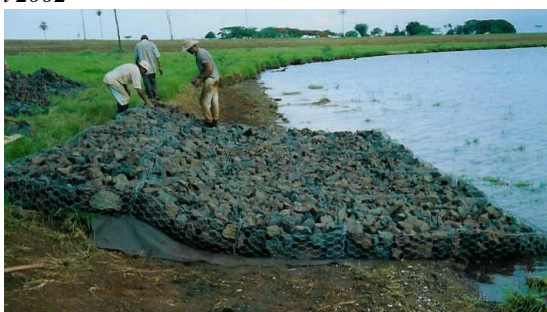
Figure 3a. Implementation of Gabion Mattress in 2002
