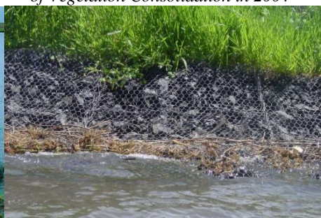
Figure 3b. Gabion Mattress at Beginning of Vegetation Consolidation in 2004
