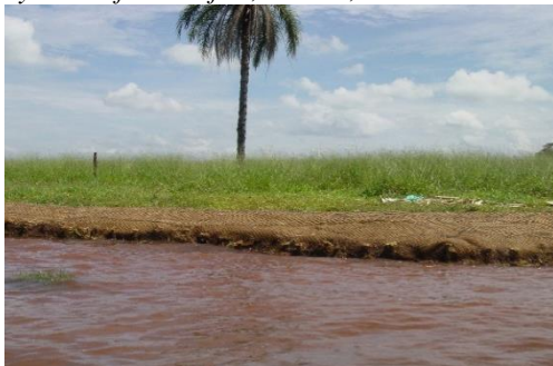
Figure 1a. Coconut Fiber Biologs Covered by RECP from Deflor, at Pier, in 2002
