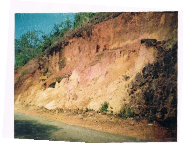
Photo 1. Land Slides and Newly Exposed Surface to Erosion
