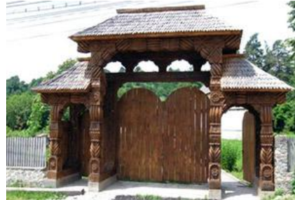
Figure 11. Traditional Wooden Gate
