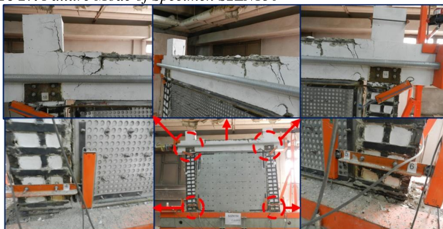
Figure 17. Failure Mode of Specimen S2ZN150
