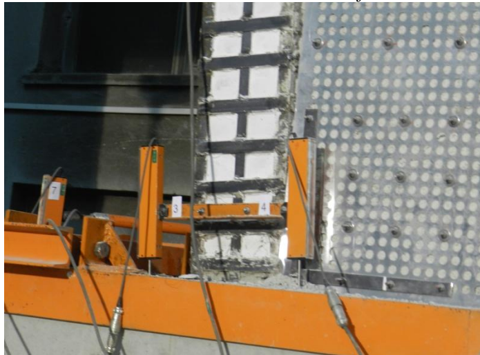
Figure 5. Rotation Measurement at the Lower End of the Column
