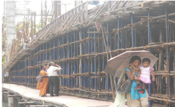
Figure 5. Shuttering System for Deck Slab and Bottom Chord of the Trussed Arch
