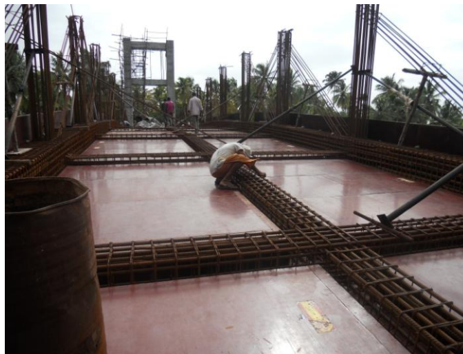
Figure 6. Reinforcement Work for Longitudinal and Cross Beams
