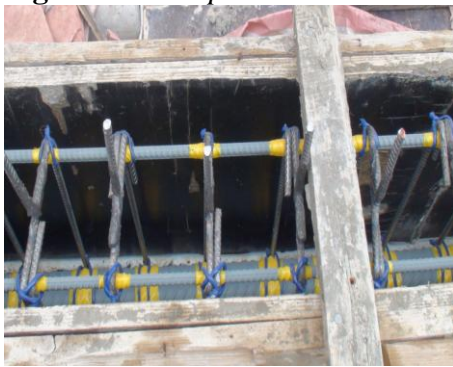
Figure 2. Stirrup Electrical Connection
