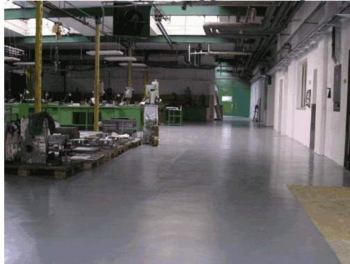
Figure 1. Example of an industrial floor applied in a production hall ([1])
