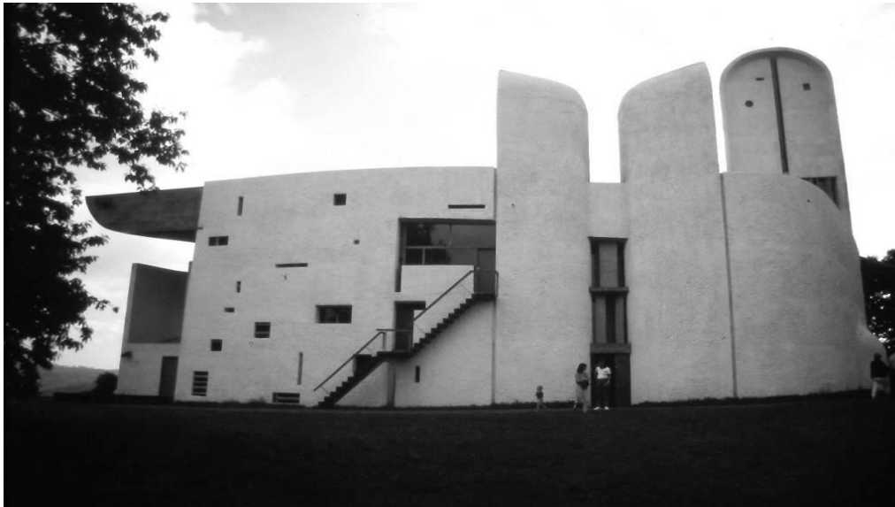
Figure 6. Exterior View of Notre-Dame-du-Haut (1950-55) in Ronchamp, France. Le Corbusier
