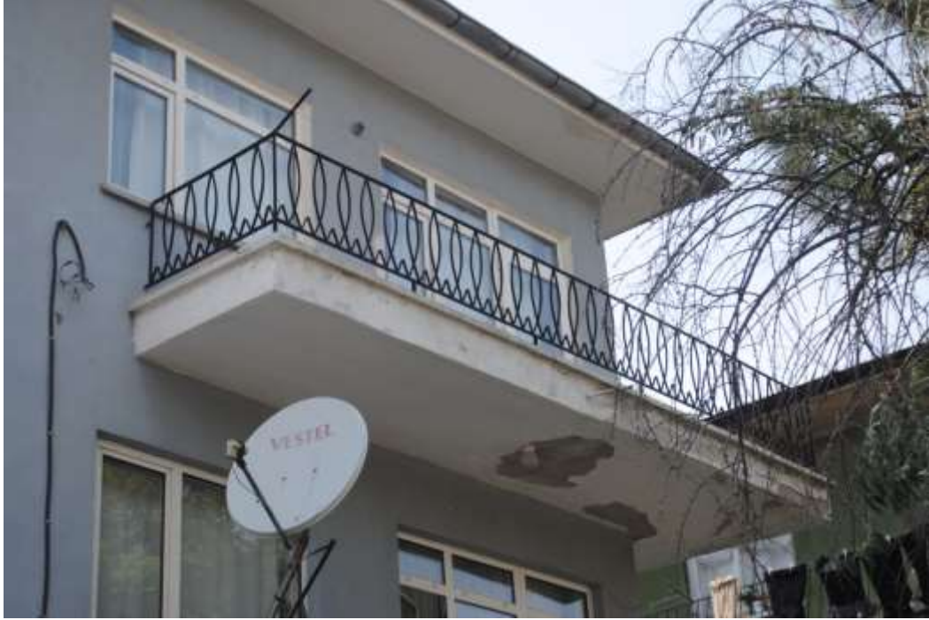
Figure 3. Ankara Balcony Railings, District 1 (Emek)
