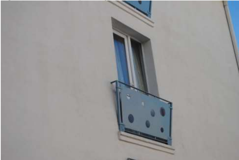
Figure 6. Ankara Balcony Railings, District 4 (Esat)
