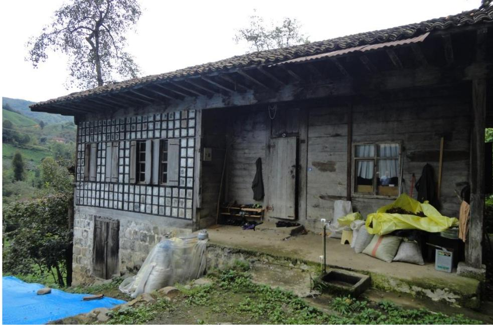
Yaşar Alişan House (Figure 20) and Orhan Tüfekçi House (Figure 21) have different construction systems from the others. Some parts of the ground floor walls of Yaşar Alişan House are cell-filled below the window sill and wooden board-filled above the window sill.
