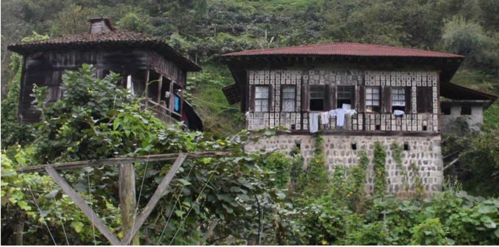
Cahit Kitapçı House (1770) (Figure 18) is the most important house in Hara Village. This is because the house is the only one with original compressed earth floor in the *aşhane*, and original wooden slats on some of the windows. These slats, used inside the wooden shutters before flat glass became common in the region, have been preserved on the east side of the house.
