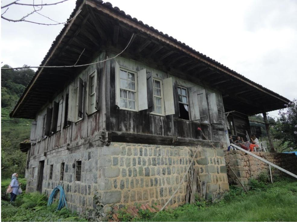
The house was constructed as timber-frame filled with wooden boards, on a stone masonry foundation and basement floor wall. In the plan, the house shows the characteristics of the vernacular plan type, and it is about the same size as Köseoğlu House.
