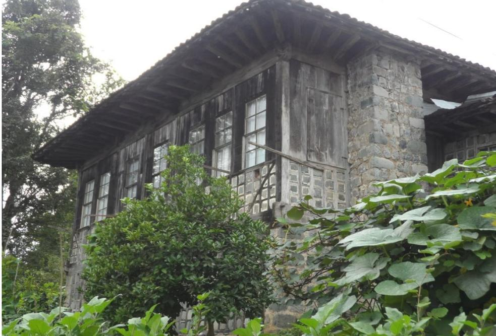
The owners of Orhan Tüfekçi House said that the house had been constructed while they were struggling with economic problems. Because of that, the construction process had taken years, and different materials had been used. The basement floors are stone masonry and cell-filled, while the ground floor walls are variously cell-filled, wooden board filled and *çakatura*.
