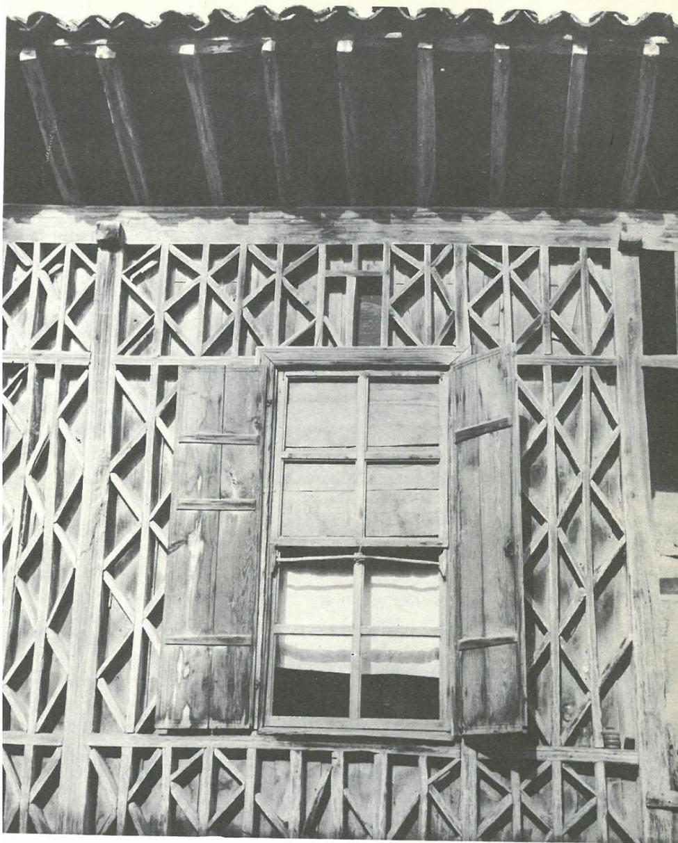
**Figure 11.** *A House with Cakatura Construction Technique in Saat Village, Fındıklı, 2014*
