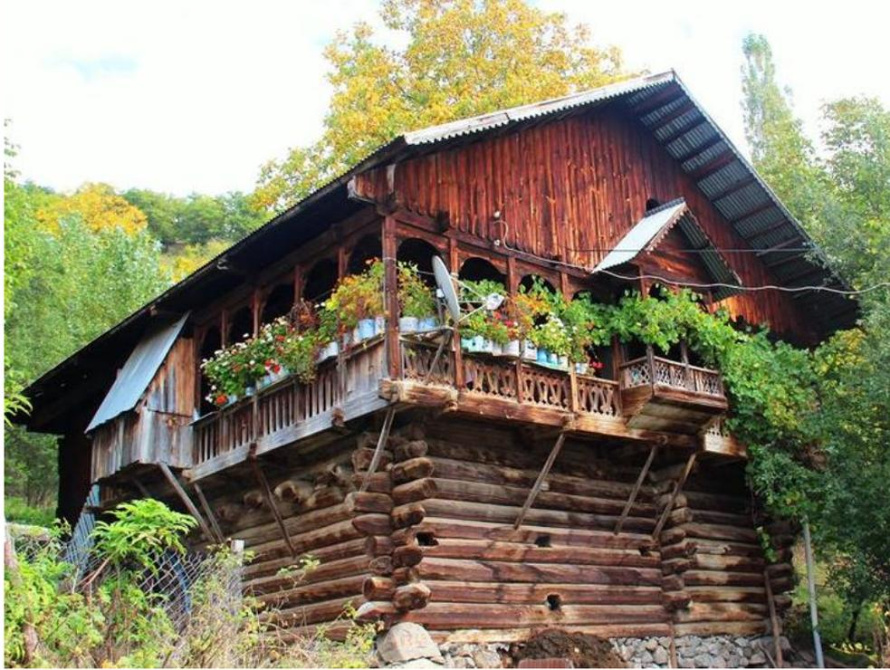
In Timber Masonry System, horizontal timber boards or timber beams are put on a stone masonry foundation and basement floor wall. These timber pieces are joined at the corners using two special nailless techniques, known as *boğaz geçme* (Figure 5) and *kurt ağzı* (Figure 6).
