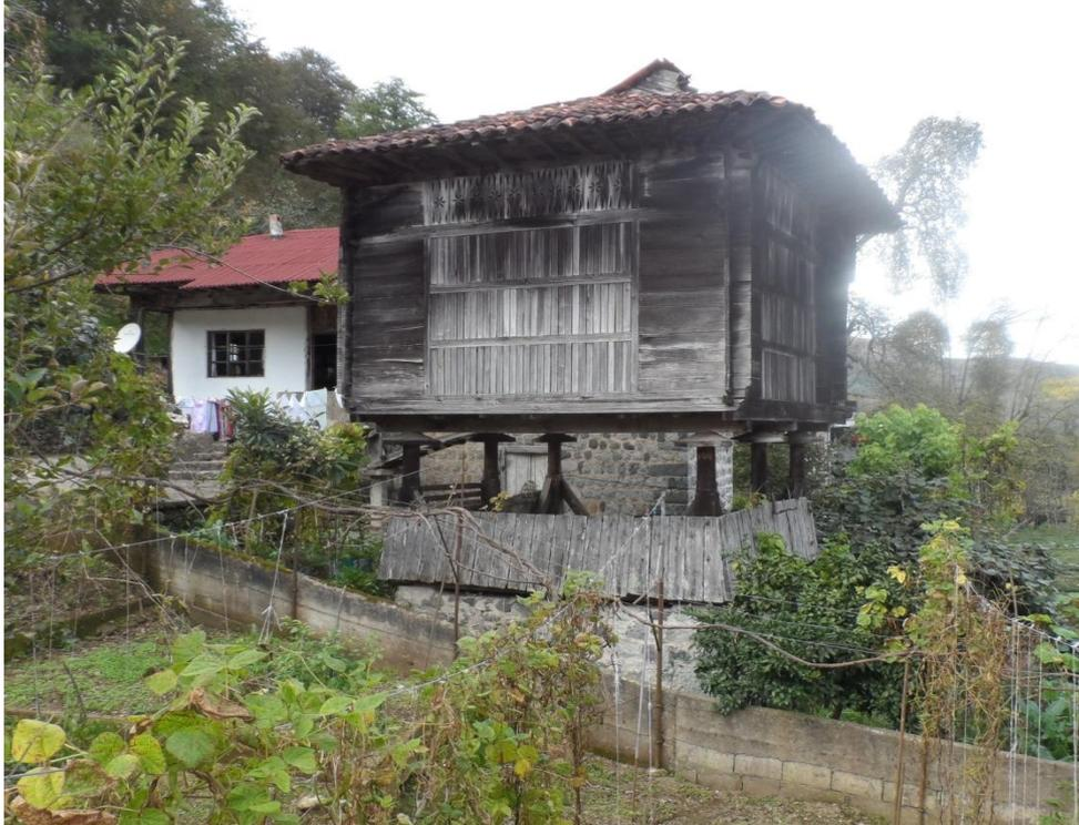
In this system, longitudinal hollows are carved into the posts, and wooden boards 2.5 to 6 cm thick, 25 to 35 cm wide are aligned between two posts along the hollows. These boards are attached to each other with wooden tenons (Figure 9).
