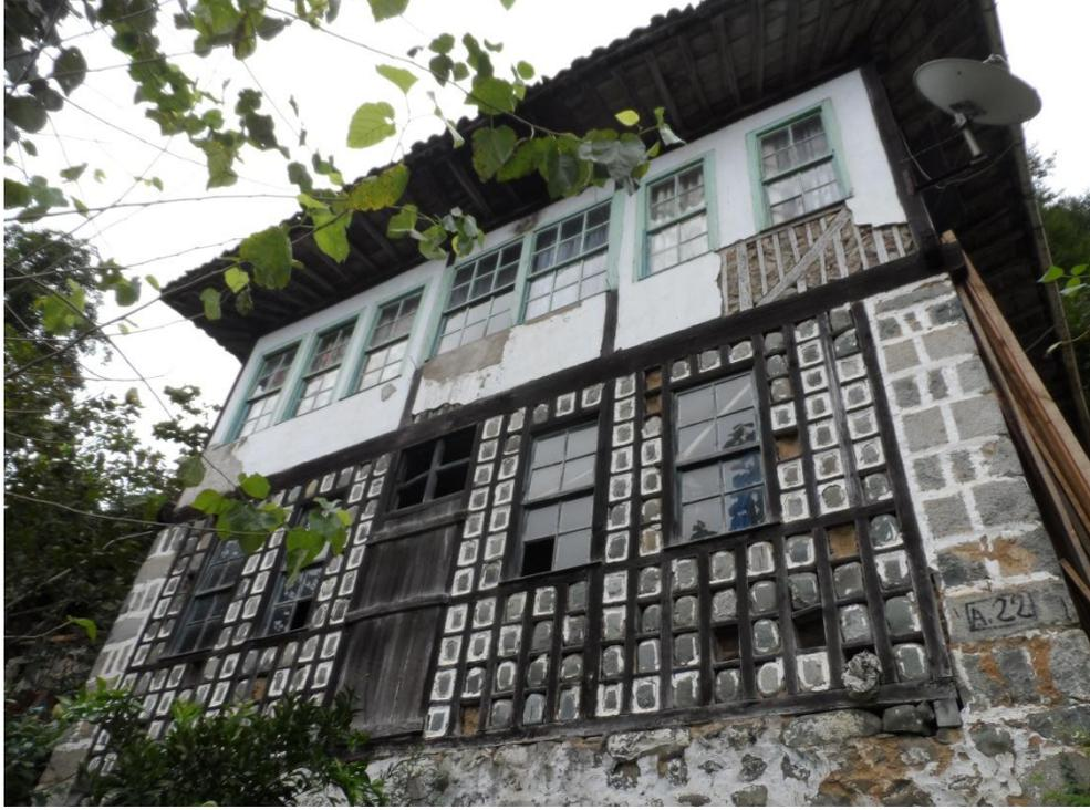
*Çakatura* is a construction technique that is disappearing because it is vulnerable to deterioration. In Hara Village, it is seen only in Orhan Tüfekçi House. An abandoned *çakatura* house (Figure 11) was observed in Saat Village in Fındıklı.
