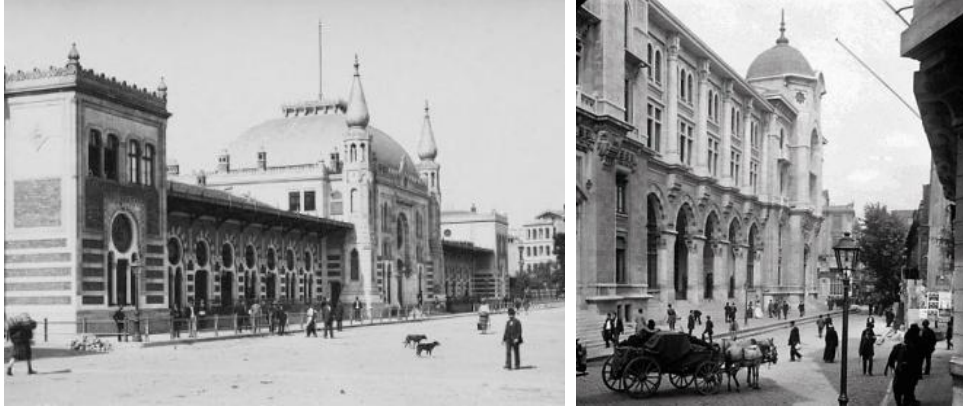
Figure 5. Sirkeci Railway Station-1890 (left) and General Post Office-1909 (right) 11
