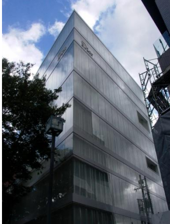
Figure 5. Sejima, Dior, Tokyo, General View
