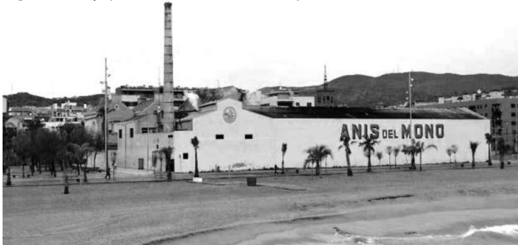
Figure 4. Sea façade. Landmark towards Seafront
