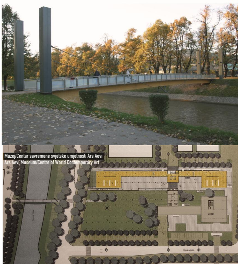
Figures 6, 7. Built Footbridge ARS AEVI; The Situation of the Future Ars Aevi Museum and the Pedestrian Bridge
