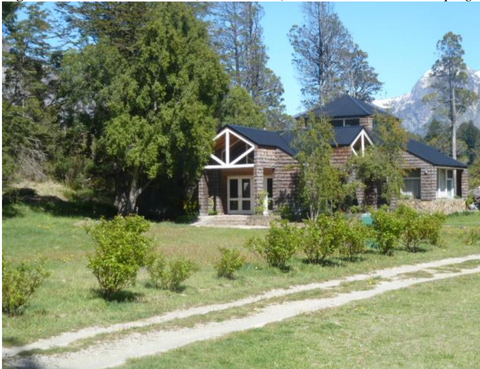
Figure 6. Rautenstrauch Hall (built in 1988), Bariloche Musical Camping
