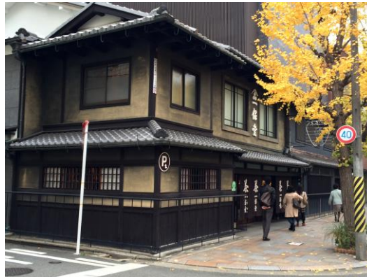
Figure 12. Modern “Machiya” in Kyoto are Restored for Public Uses such as Tea Houses, Hotels, Shops, Galleries, Museums or Community Centre. / Credits: Authors
