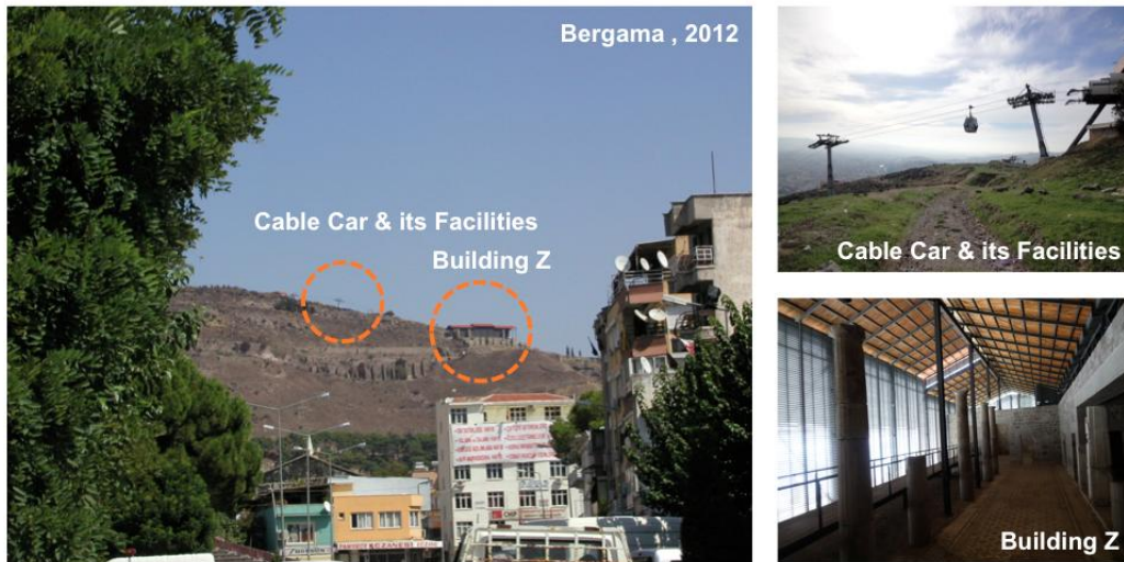
Figure 8. Building Z (A Site of Archeological Remains), Cable Car and Related Infrastructures on Acropolis Drew Public's Attention and Discussion on Urban Landscape Preservation. / Credits: Authors
