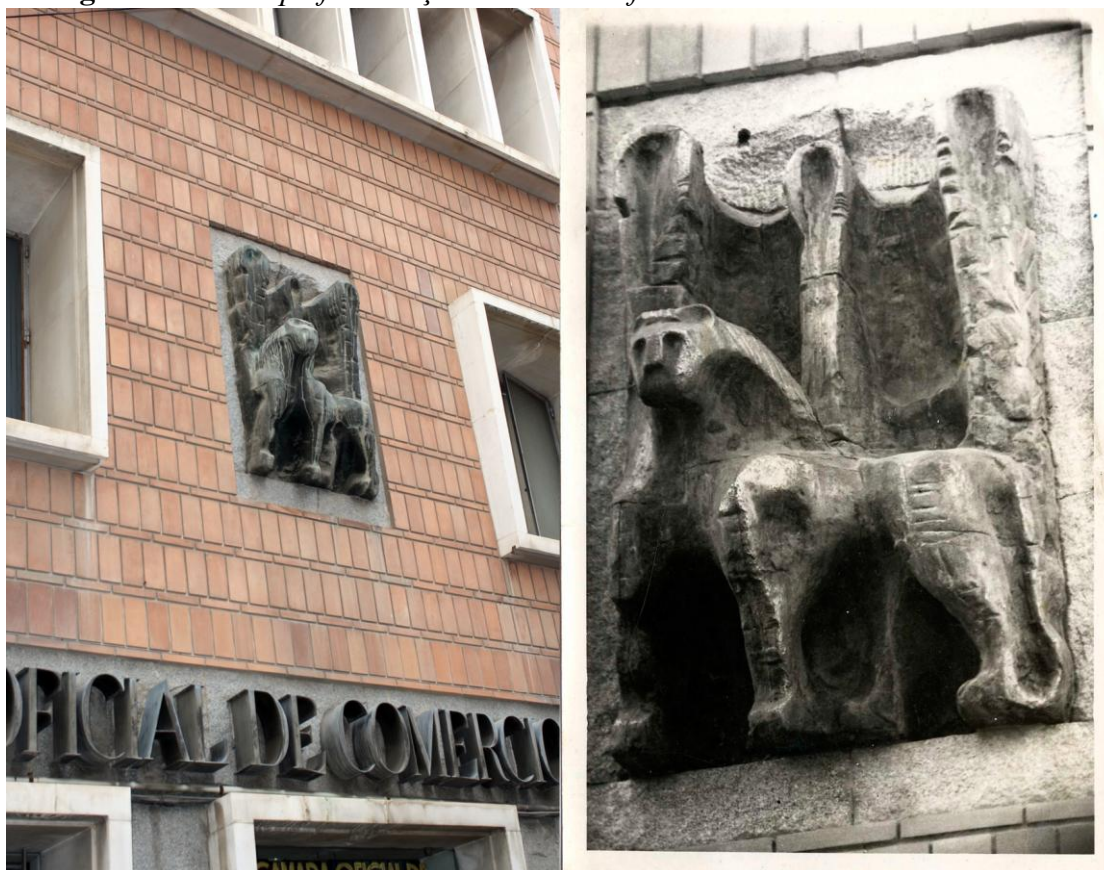
Figure 2. Close-up of the Façade and Coat of Arms
