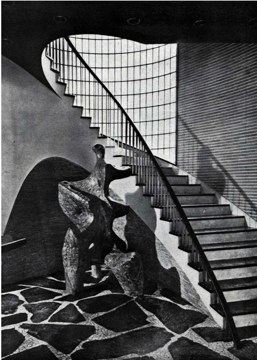
Figure 7. The Staircase and Oteiza's Sculpture on the Ground Floor (1955)
