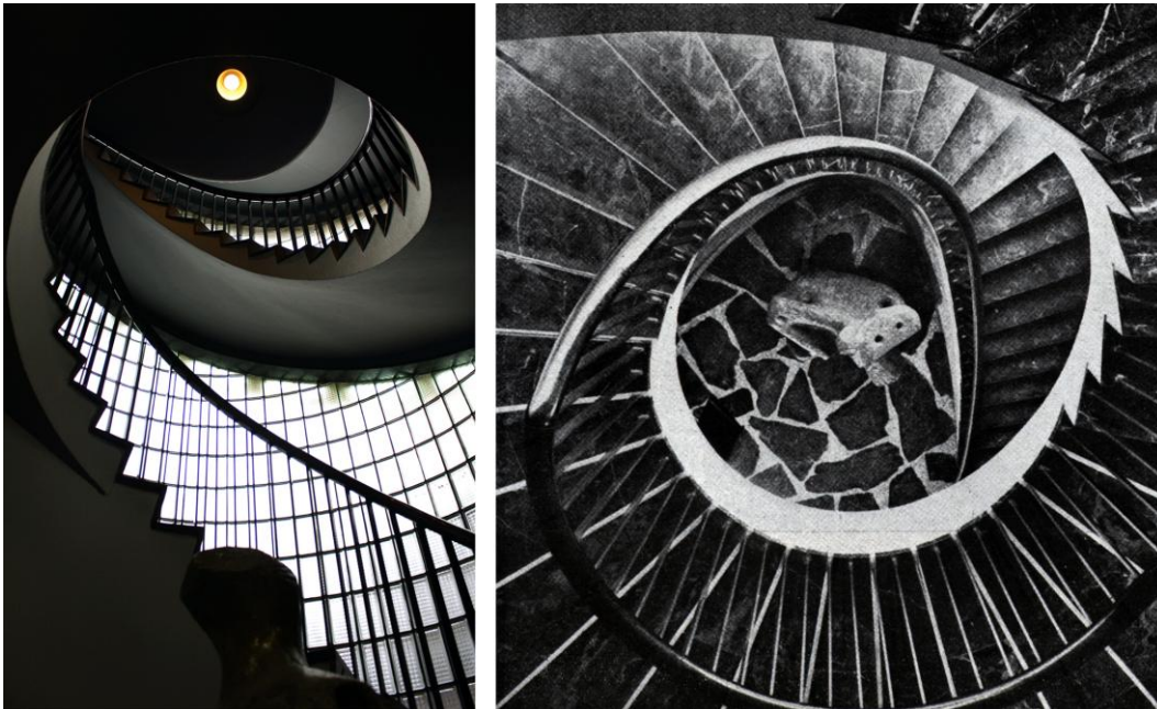
Figure 9. Left: Stairwell seen from the Ground Floor (1955). Right: View of the Stairwell from the Second Floor. The Paving on the First Floor Imitates an Infinite Staircase (January 2011)
