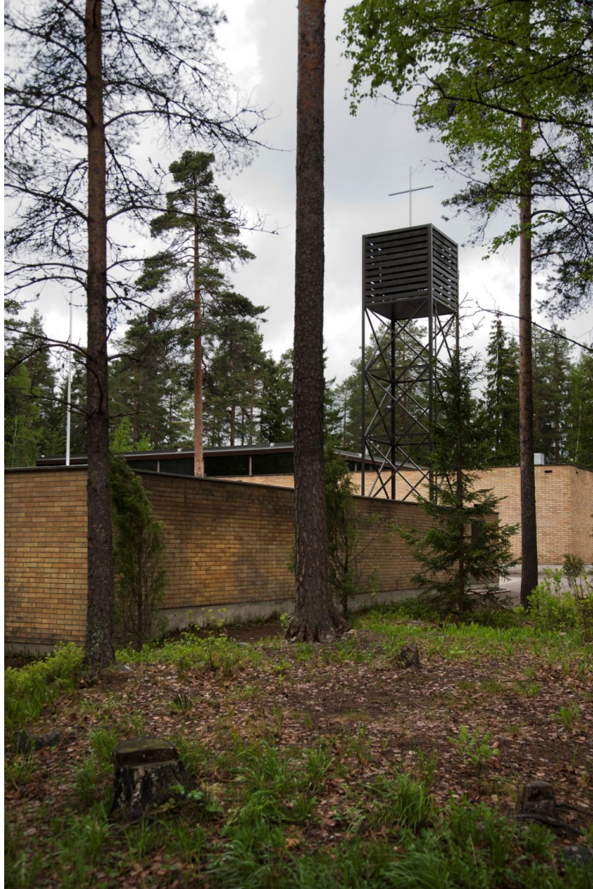
Figure 5. The Salpausselkä Church by Architects Woldemar Baeckman and Helmer Löfström. Photo Tiina Rekola / Lahti City Museum Photograph Archives
