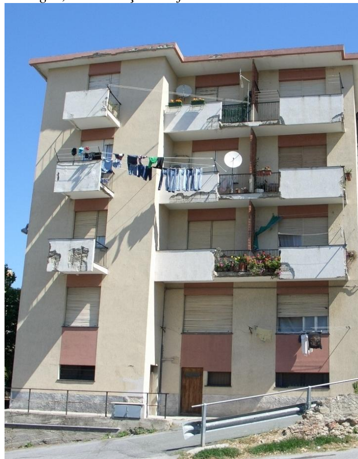
Figure 3. Building C, South Façade before Renovation
