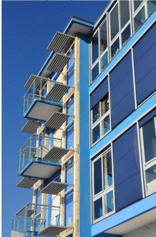
Figure 6. Building B, South Façade after the Retrofitting
