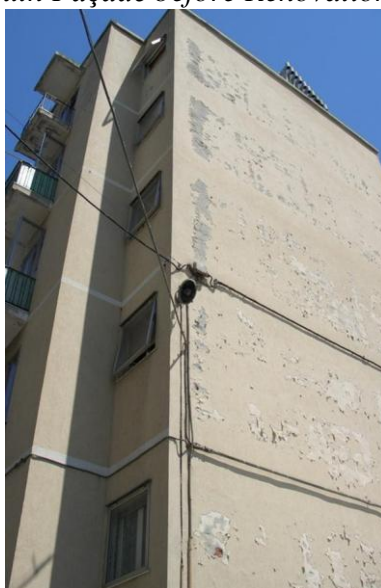
Figure 1. Building A, South Façade before Renovation
