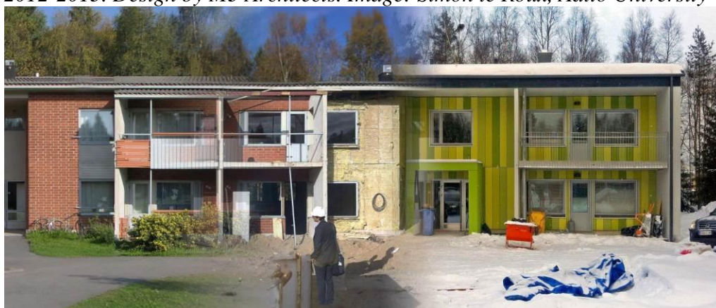
Figure 7. Panorama Showing Case Virkakatu Before, During and After Retrofit. Year of Building: 1983. Size: 2-Storeys, 8 Rental Apartments. Retrofit: 2012-2013. Design by M3 Architects. Image: Simon le Roux, Aalto University
