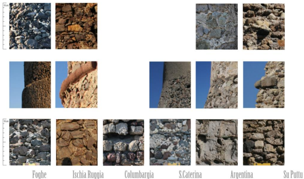
Figure 4. Details of Masonry Referring to Some of the Towers Investigated. The Comparison Highlights the Different Masonry Textures that Characterize the Basis and the Upper Body of Each Tower and the Constructive Solution Adopted for the Connection between the Two Bodies. Graphic Realization: S. Murru
