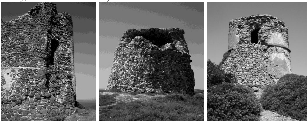
Figure 6. Foghe, Su Puttu and Iskra Ruia Towers. All These Examples Are in Bad Conditions, because Neglected. All the Images Put in Evidence the Various Questions of Degradations, i.e. Erosion, Alveolization, Anthropical Decay, Structural Instability. Photos: S.M Grillo
