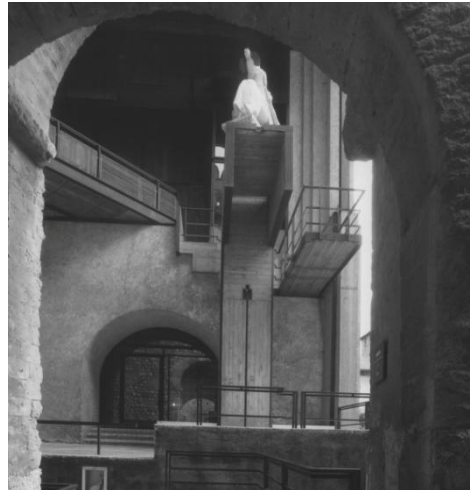
Figures 3-4. Steel fragments in Castelveccchio Museum: architectural detail of the metal beam and the walkway
