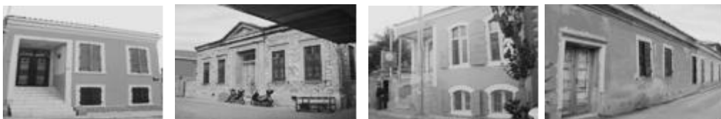
Figure 1.1. An example of an elevated basement storey house without bay windows and with an entrance on one side placed into the niche. Figure 1.2. An example of an embedded basement house with an entrance in the middle placed into the niche. Figure 1.3. An example of an elevated basement storey house with an entrance through the platform. Figure 1.4. An example of a one storey house with a wide front.
