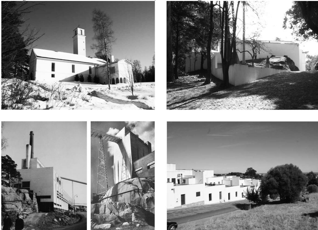
Figure 2. Aalto's Muurame Church (1926) and Sunila Pulp Mill (1935-39), on the left | Siza's Quinta da Conceição Swimming Pool (1958-65) and Malagueira Residential Area (1977-...), on the right
