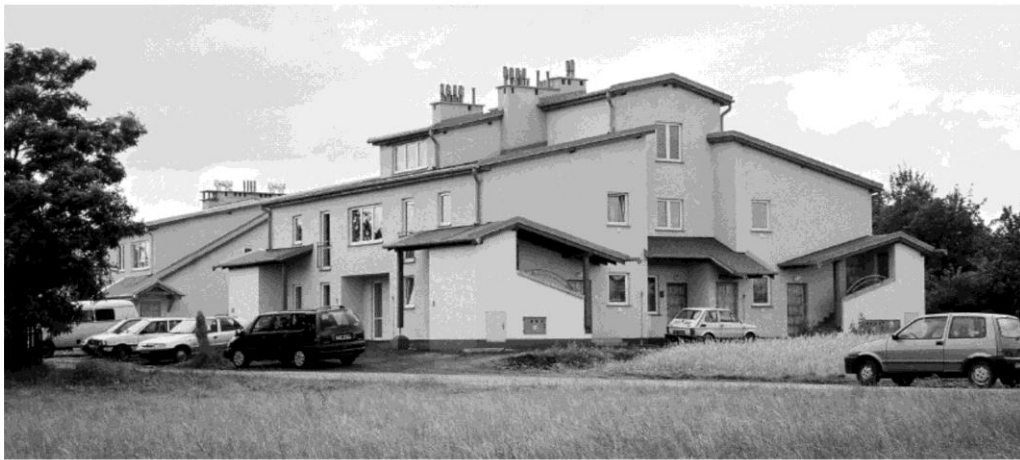
Figure 4. Stacked six-plex in Mikołów, Młyńska Street, architects: Jan Pallado (chief designer) and Aleksander Skupin, a - ground floor, b - first floor, c - second floor, d - section, e - photo (J.Pallado)
