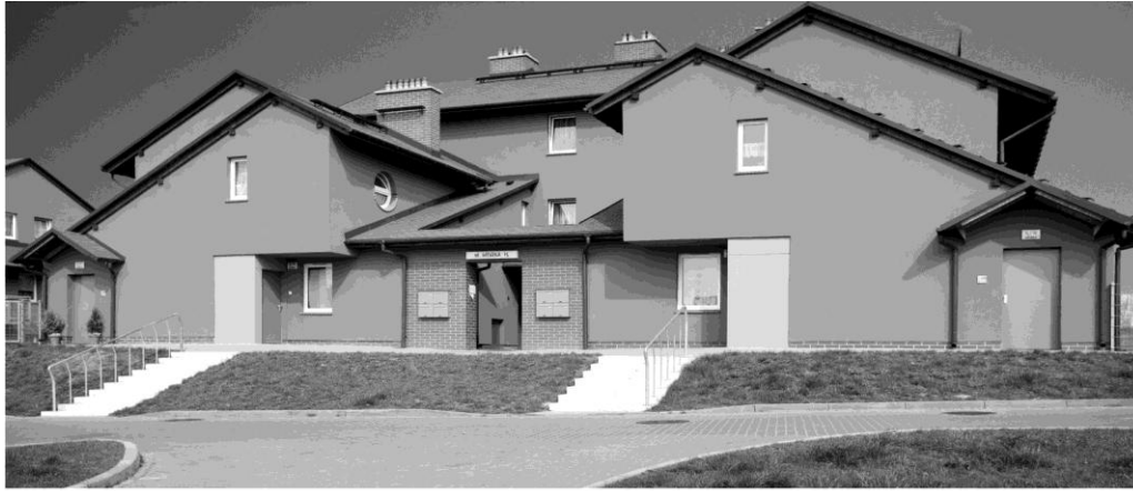
Figure 5. Stacked eight-plex in Ruda Śląska, Cynkowa Street, architects: Jan Pallado (chief designer) and Aleksander Skupin, a - ground floor, b - first floor, c - second floor, d - section, e - photo (S.Polański)
