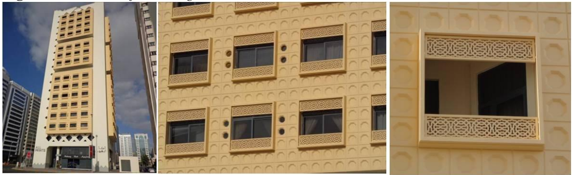
Figure 1. Sheikh Seif Building Abu Dhabi
