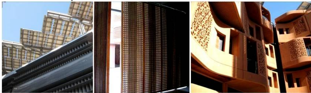
Figure 4. Masdar City: metal, wood and GRC Screens
