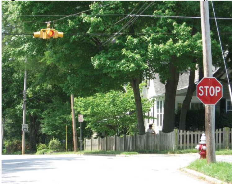
Figure 1. Intersection Standard Overhead Flashing Beacon
