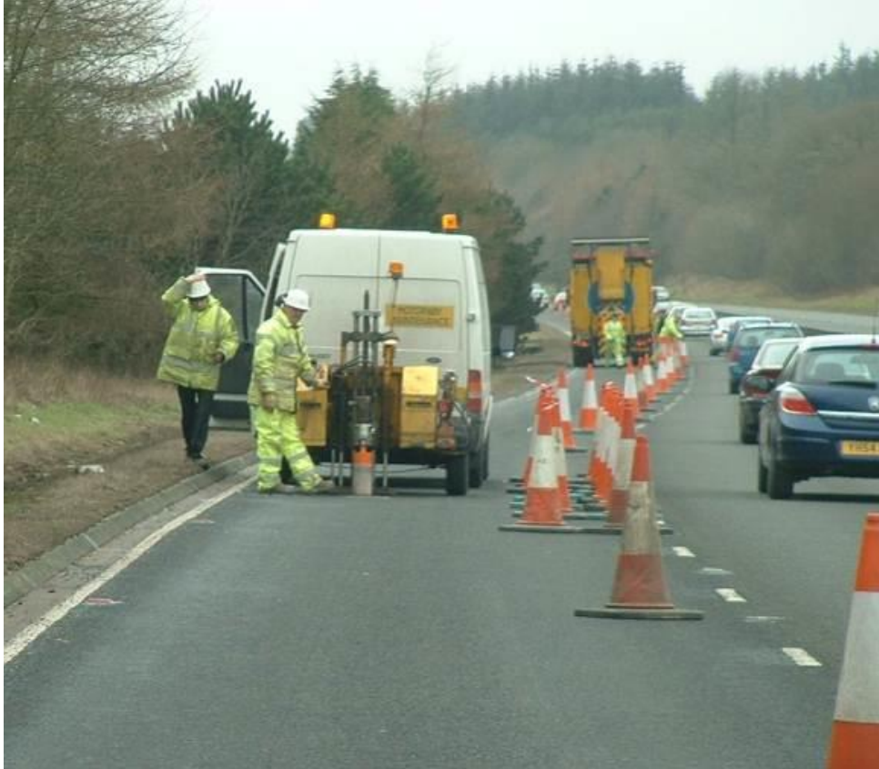
Figure 2. Extraction of Asphalt Core Sample Used from Asphalt Pavement
