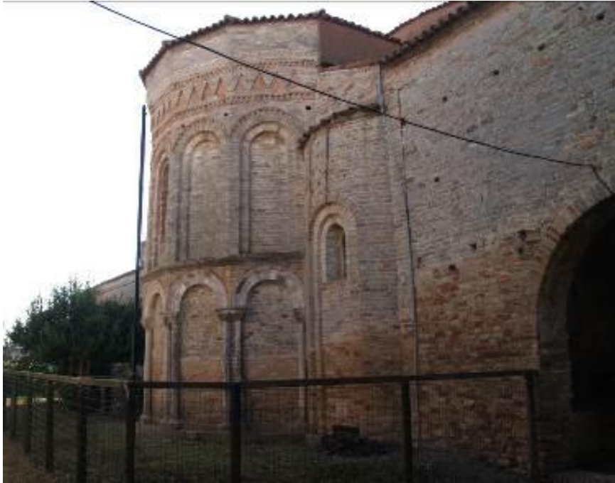
Figure 3. Eastern External View of the Church
