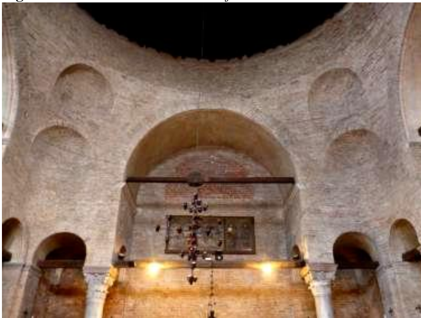
Figure 2. Northern Internal View Of The Church
