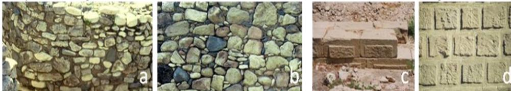
Structural reasons and especially the need for stability led the traditional builder to the erection of thick stone and mud brick walls of 50cm. At the same time the thickness of the wall has an interesting aesthetic result. The
