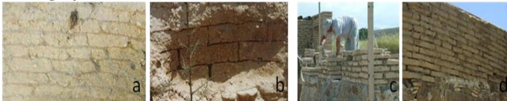
Similar methods of dressing and erection of stone walls have been used diachronically (Figure 2). Most of the walls followed the shell type building system with ashlar or large rubble stones used for the exterior faces of walls. A common characteristic of ashlar walls was the dressing and smoothing of only the faces that were meant to be visible and partly of the surfaces set against other stones leaving the back of the stone unworked (Philokyrou 2011).
