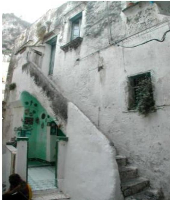
**Figure 5.** *Fjord of Crapolla, Detail of rural houses' masonry. It's possible to see the simple constitution of wall made by local material*
