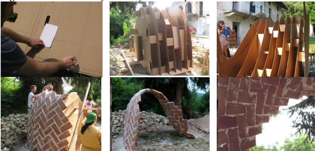
**Figure 17.** *Sequential Steps of Formwork Construction*
