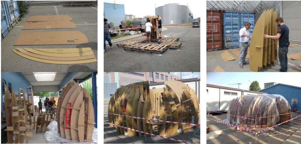
**Figure 19.** *Sequential Steps of Construction*
