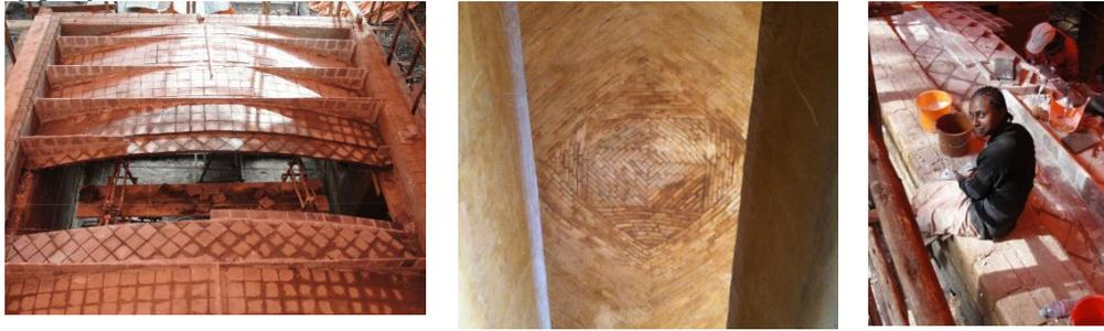
**Figure 10.** (a) *Free form vault (Davis, 2012); (b) Formwork of Free-form vault (Davis, 2012); (c) Structural test over the Free Form thin-tile vault (Davis, 2012)*
