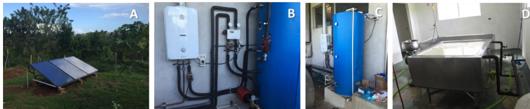
Figure 5. Thermal Hybrid Forced System Implemented at LLAFRAK and San Bosco Dairy Factories (A) Solar Panels (B) Auxiliary System (C) Reservoir for Hot Water (D) Solar Cooking Pot for the Pasteurization of Milk
